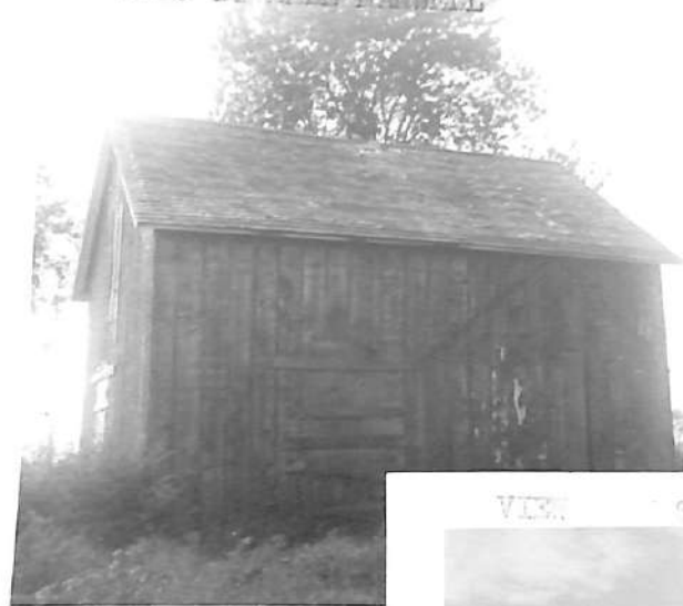
VIEW FROM EAST SIDE
