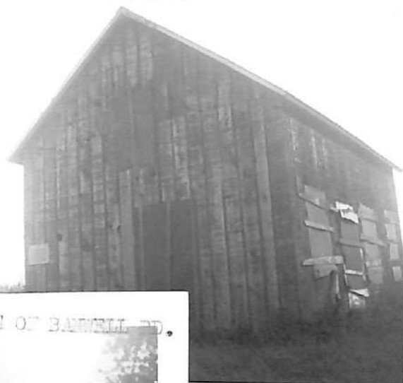
VIEW FROM NORTH SIDE - BANWELL ROAD
