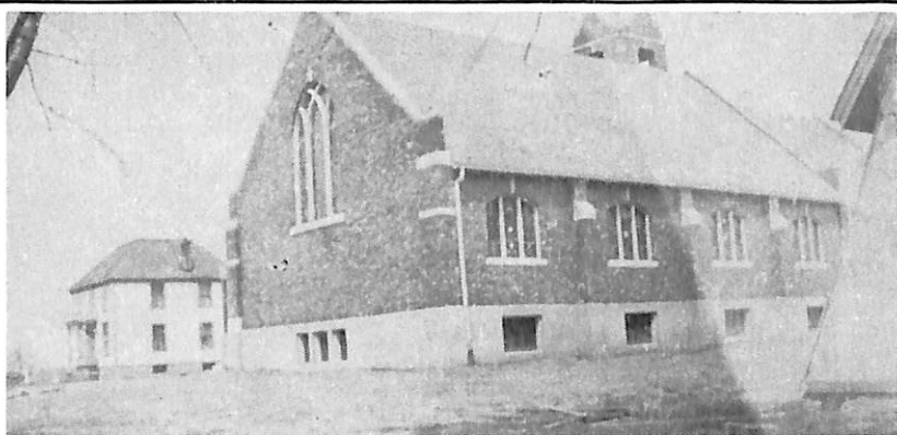
October, 1913 showing the old church in the right hand corner, new church and the rectory moved to the new site.
