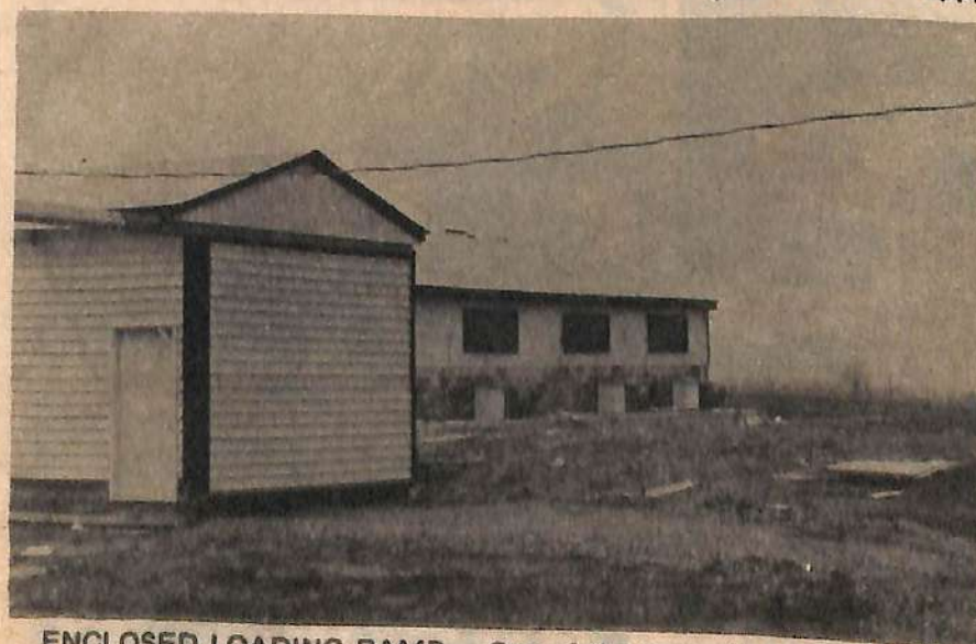
ENCLOSED LOADING RAMP -- One of the innovative ideas Ted Ure had for his new hog finishing barn was an enclosed loading ramp (as seen in foreground). Ted said the ramp would be more efficient than the conventional open one. Air vents for the eight-foot-deep manure pit can be seen at the side of the barn. (Staff Photo -- P. Epp)
