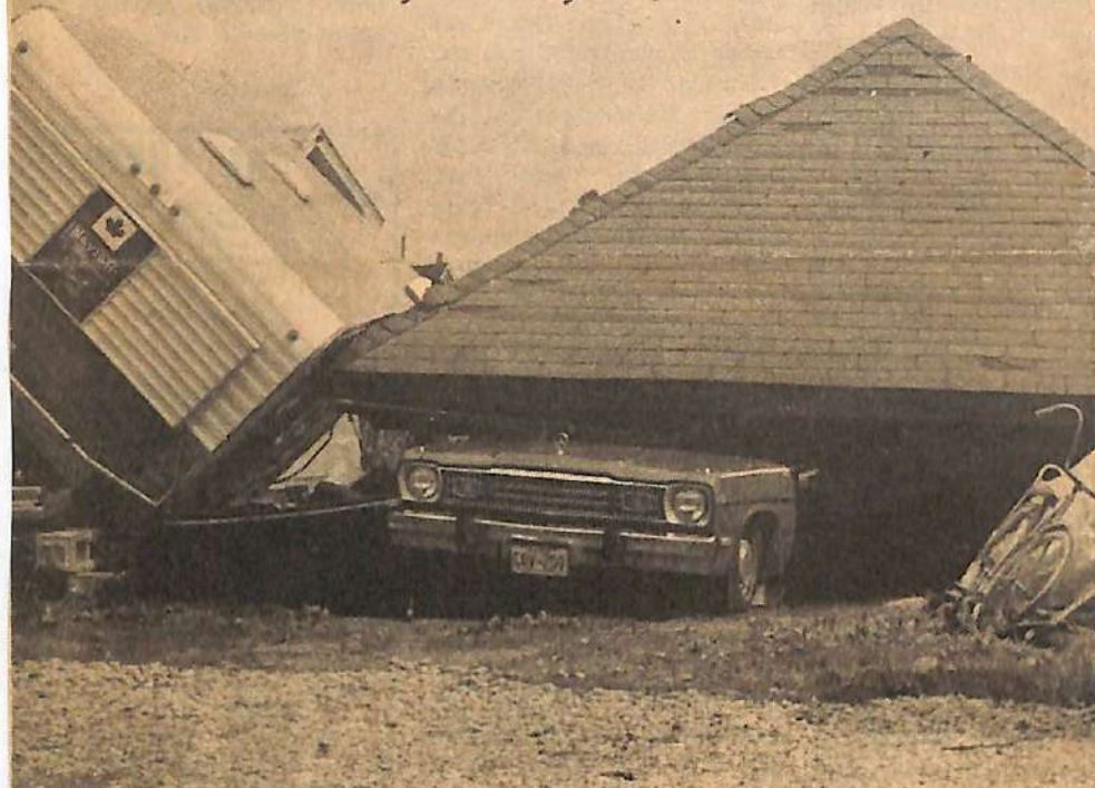
Tuesday night's wind knocked the cement blocking right out from under this garage belonging to Mark Ganzer on the 9th concession of Sandwich South. The trailer camper was blown over and it hit the garage.
