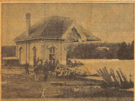
The old pumphouse at Springbank just west of London, as it-looked in the year 1883 after a flood had surged down the Thames River, taking a mighty bite out of the building. The PUC pumphouse, however, was made of enduring material. was rebuilt, survived another flood in 1937 and still is standing with the original section, seen here, housing present-day pumping equipment.
