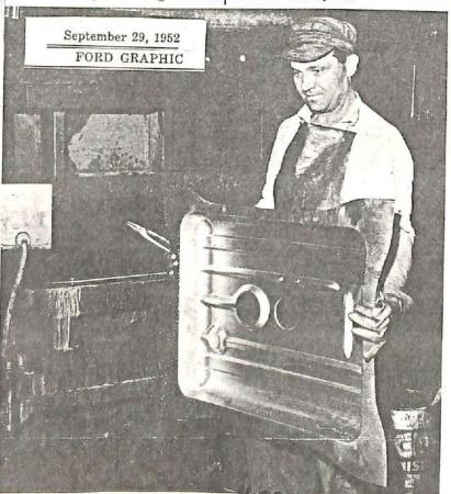
(b) On the other side of the press, Con Daniger removes the sheet. It has now been formed into a half section of a gas tank.
