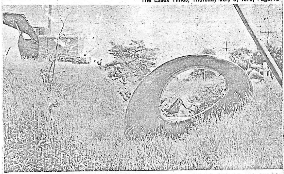
"SOMEBODY SQUASHED MY DRAIN PIPE" Not really, it's supposed to look like that, say the contractors. The 56 foot long multiplate culverts are being installed at the junction of the 8th and 9th concession, Sandwich South and Town Line Road. The county states that the narrow bridges were a hazard to wide-turn vehicles such as school buses. The tab, which the county picked up was $6,275 and $6,965 for the two jobs.
