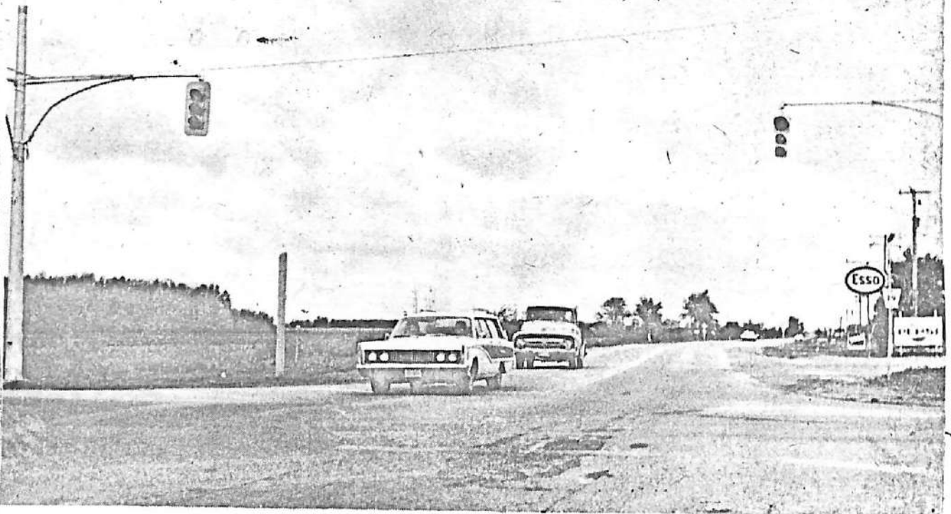
NEW STOP LIGHTS. Traffic lights were installed last Friday at the intersection of Essex road 19, and County road 46. At present the lights were left flashing red for north and south bound traffic on Essex road 19 and flashing caution for east and west traffic on County road 46, until drivers become aware of the lights.
