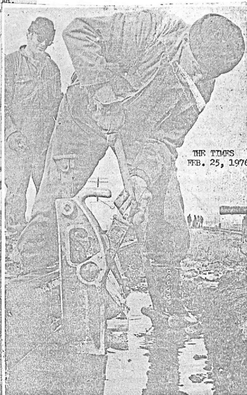
BETTER MUDDY THAN ICY? — Walt 'Woodpecker' Woods works in the muddy waters of the Walker Road railway tracks. He and Fred Hoffman were part of a maintenance gang shimming up the tracks with plywood strips. Although the ties were still frozen, the upper crust had thawed and no ice chipping was necessary. Usually the ties are raised, and gravel put underneath but with the frozen ground, the shims were necessary. As soon as warm weather comes to Essex County, they will probably have to be taken out.
