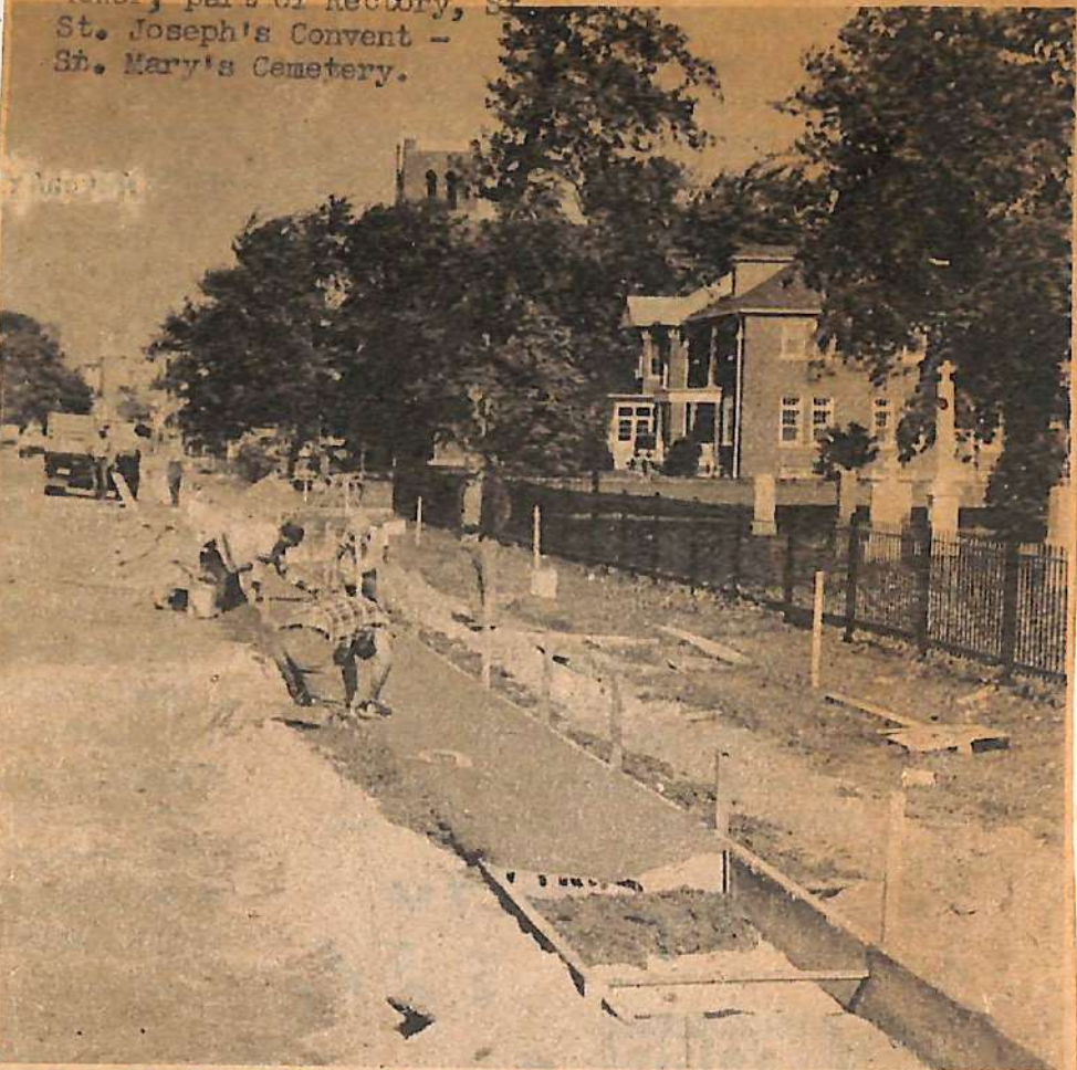
REPAIRS IN MAIDSTONE — Crews of the Ministry of Transportation lay curbing along No. 3 Highway from the intersection in Maidstone to the east edge of St. Mary's Cemetery after installing storm sewers. A sidewalk will be laid along the edge of the curbing before the work is completed. SEP. 19, 1974 ESSEX FREE PRESS
