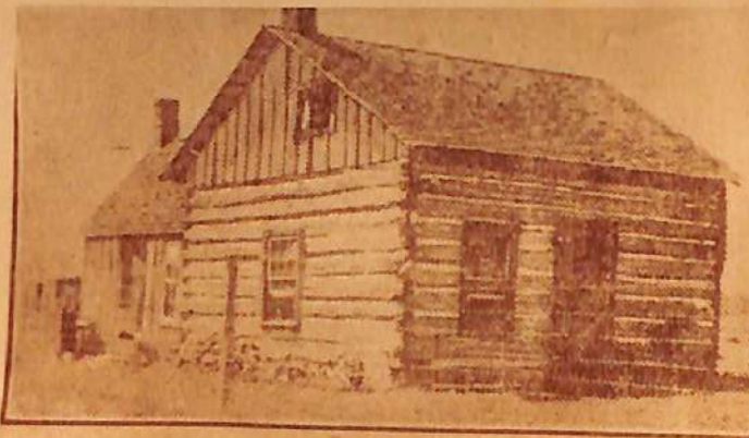
T HIS is one of the oldest log houses around the McGregor settlement. It was built by Mose Dufoe of rough-hewn logs and plaster. Although not as old as some of the other houses nearer the lake shore, this has served as a dwelling for over 60 years.
